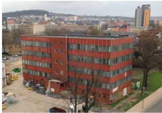
Once the central switching unit of a large company: "Tomato", shortly before it was razed to the ground in 2013.
